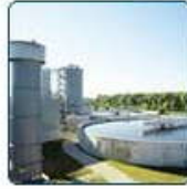
Waste Water Treatment
